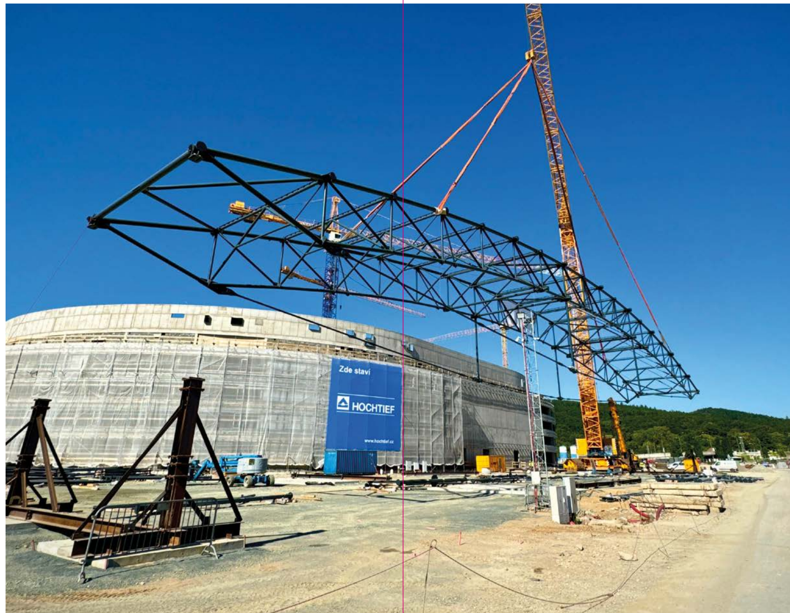
Brno, Multifunkční hala Arena Brno Brno, Multi-purpose hall Arena Brno
